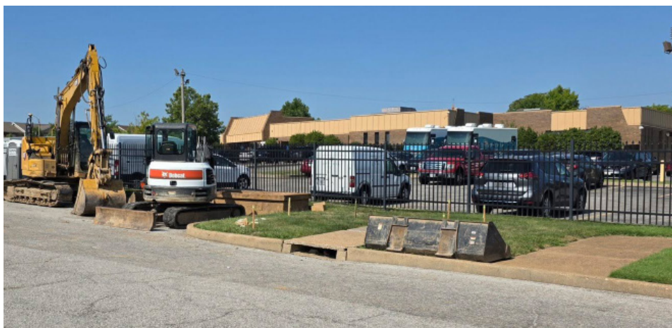
Construction beginning in early August.
